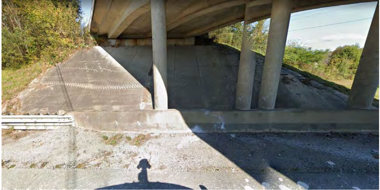
EB I-24 Looking North Under Bridge
