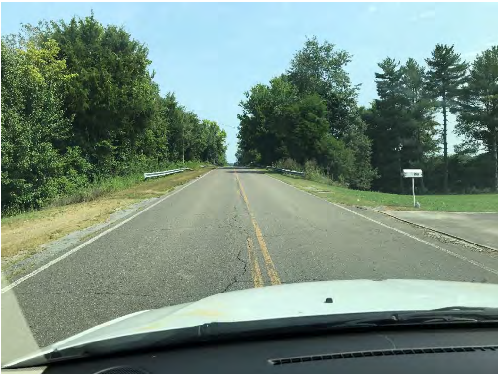
Southern Approach looking North
