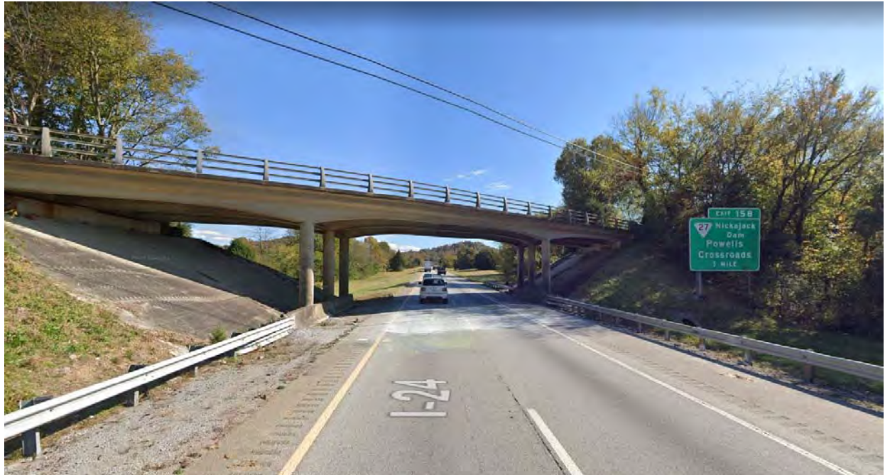
EB I-24 Looking East Under bridge
