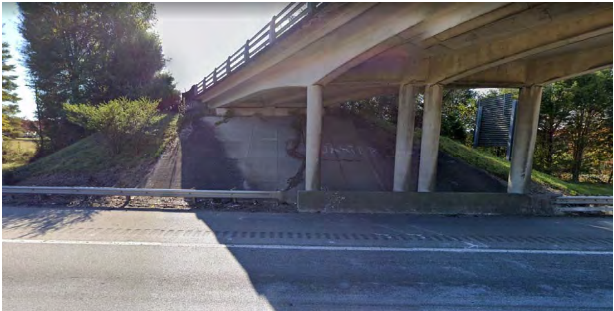
EB I-24 Looking South Under Bridge
