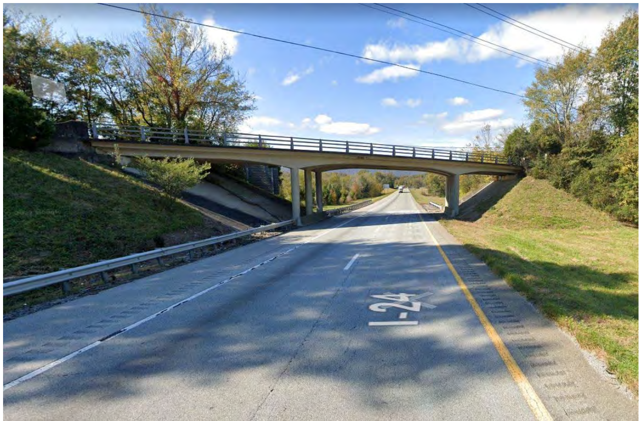
EB I-24 Looking West Under Bridge
